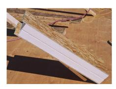
The *Insulspan*® *SIP* (*Structural Insulating Panel*) *System* is an energy efficient building system that consists of a core of *PlastiSpan*® expanded polystyrene (EPS) insulation with SIP-grade oriented strand board (OSB) structurally laminated to the interior and exterior faces of the EPS insulation core.
